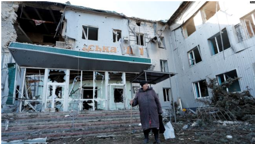
Destroyed hospital in Volnovakha , Donetsk region, March 12, 2022.
